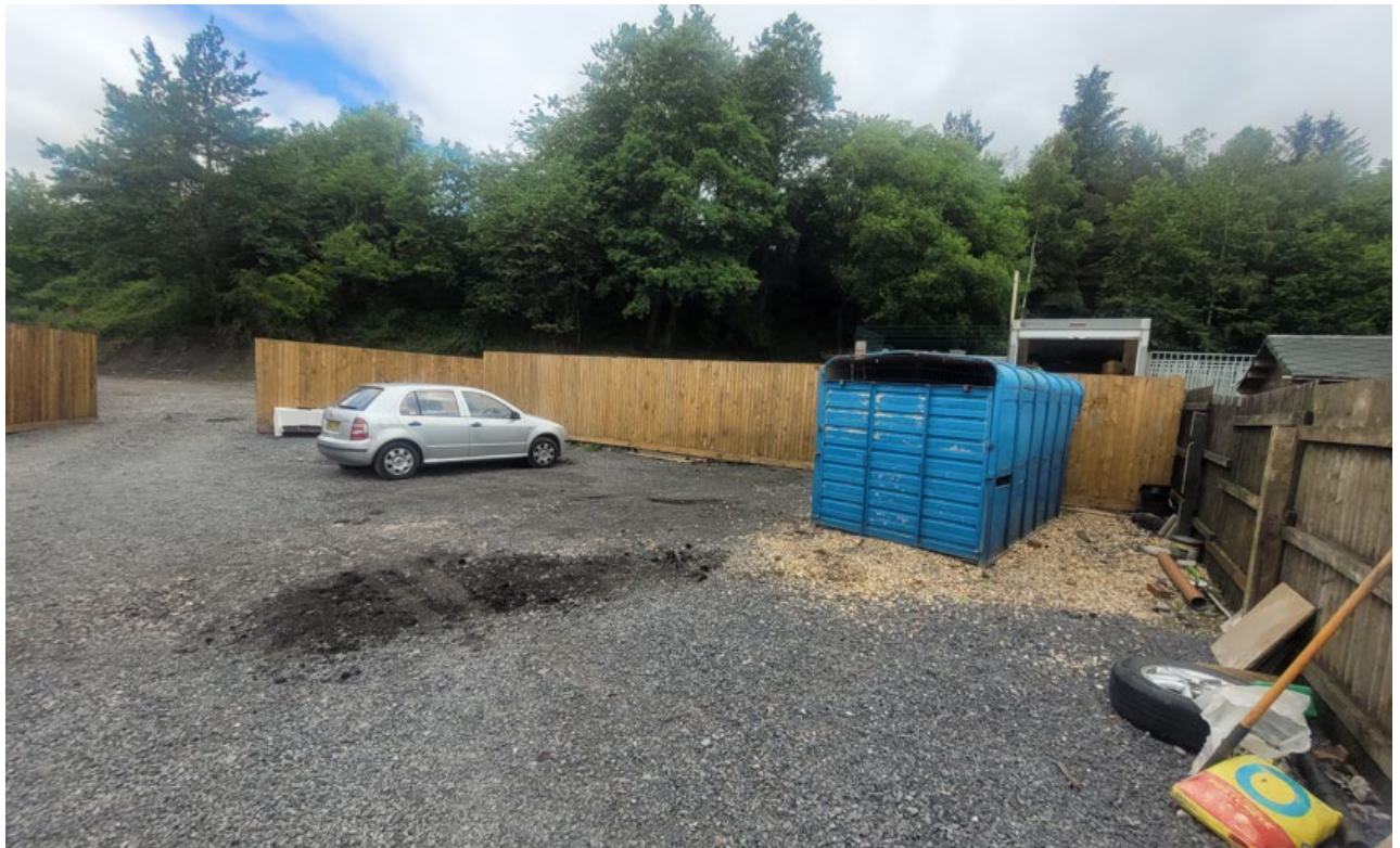
Fig 6: boundary fence erected. Gap in the fence shows an access leading to the land to the north (outside the application site).
